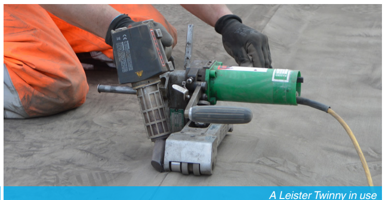
CC Hydro™ double/triple-track weld
