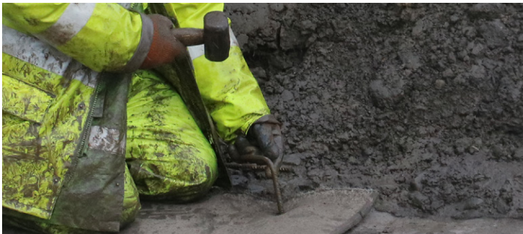
CC being fixed with a ground peg
