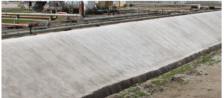
CC fixed to concrete drainage channel
