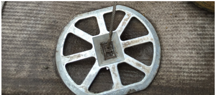
A Percussion Anchor fixed into place
