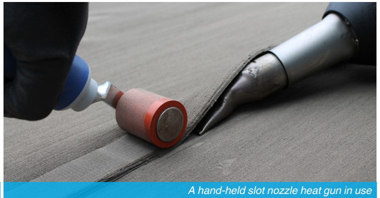
Thermally Bonded Overlap Joint
