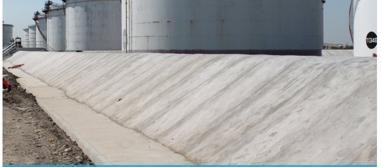
CC captured within a poured curb
