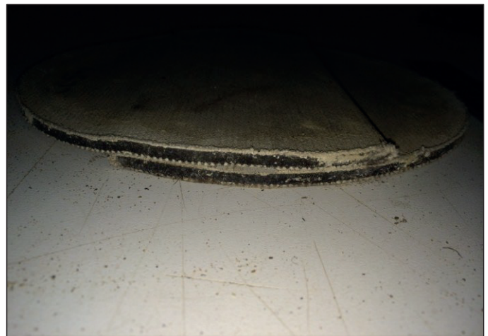
Figure 6. CC5-1 joint after the test, no root penetration
